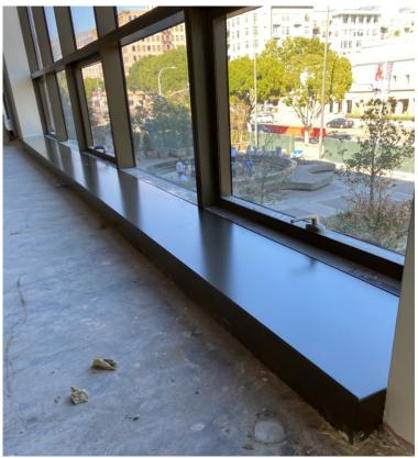
The Architect was passionate about keeping the operable windows throughout the project and leaving them down at the sill condition of each floor, which is unfortunately below the allowable ADA height. This required the Aragon team to find and install low-energy window operators that could be switch controlled at the point of use, all while maintaining this feature within the owner's budget.
