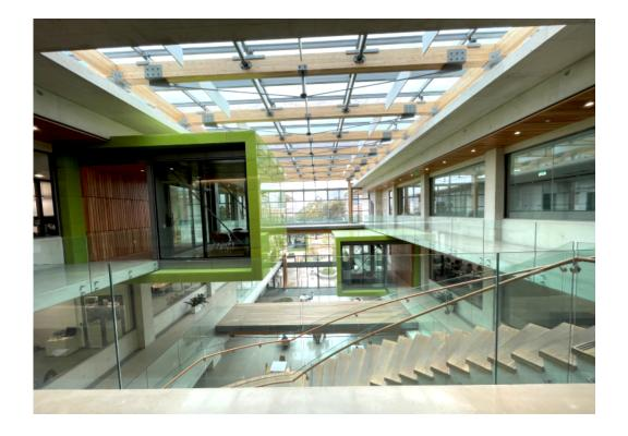
Inside and outside the atrium, Perkins & Will added meeting "pods" to encourage collaboration. The projecting pods are clad in a green accent glass clad rainscreen panel system on both vertical and horizontal surfaces. The glass panels were a series of complex shapes backed by concrete board, with a 'Z' girt clip attachment to furring channels.
