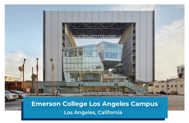
Dynamic facades, ones that not only provide for the high-performance enclosure of a building but through innovative design react to the environmental demands, are part of the continuing evolution of modern architecture. In this SCGMA Case Study, we look at a complex façade and how the integration of operable sunshades enhanced energy performance as well as greater occupant comfort.
